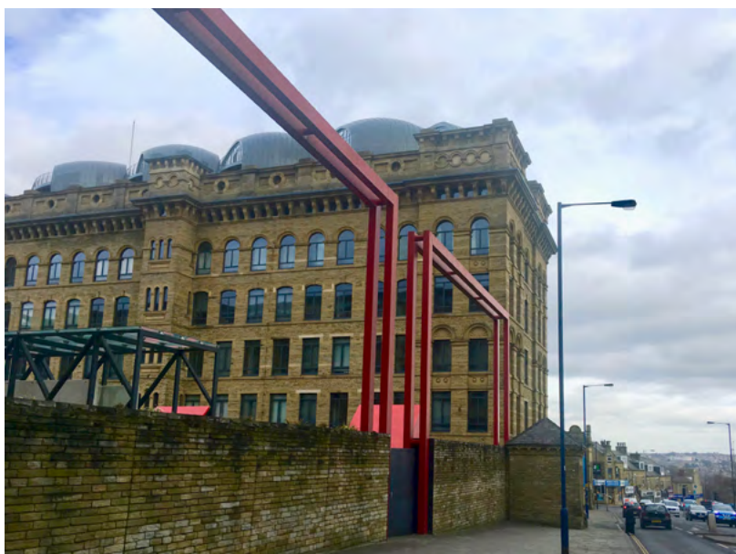
The repetitive curved and futuristic pods on top of the converted Lister Mills building demonstrates an innovative and contemporary response to the original mill building's large scale and traditional repetitive facade, which features a strong vertical rhythm of frontage, arched windows and intricate detailing particularly around the building's 'crown'.
