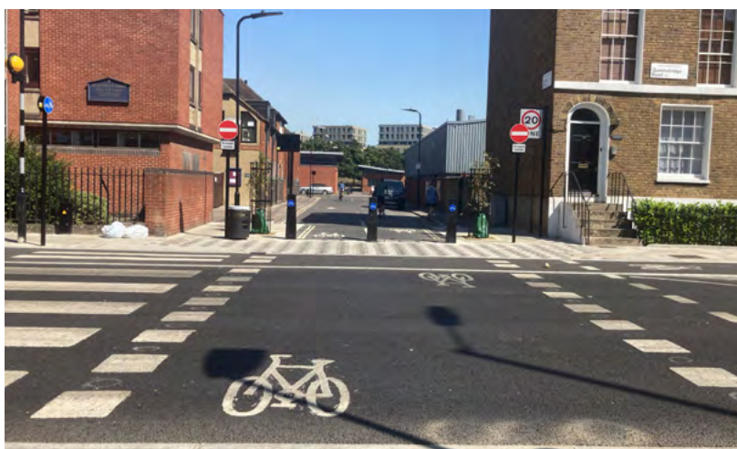
A continuous footway and bollards create a modal filter across a former vehicular junction to give cyclists and pedestrians priority.
