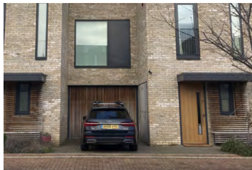
Outdoor storage is located by the front door and accessed via the on-plot parking space.
