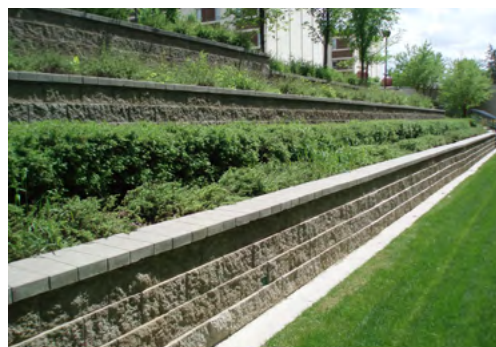
Stepped vegetated walls are an attractive solution which can contribute to achieving the urban greening factor as well as biodiversity net gain (refer A.1) (Photo © CornerStone Wall Solutions)
