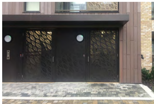
Communal cycle storage is provided for flats behind a metal screen by the entrance.
