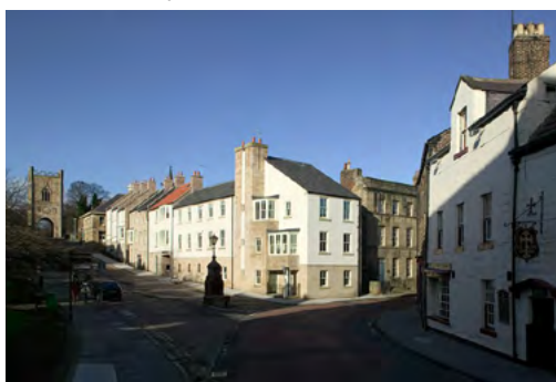
New-build flats in Alnwick, Northumberland successfully respond to the traditional local character of its surroundings without appearing pastiche by utilising a prominent chimney stack, bay windows, and similar rhythm of frontage and window proportions. (Photo © Sally Ann Norman, Architect: JDDK Architects)
