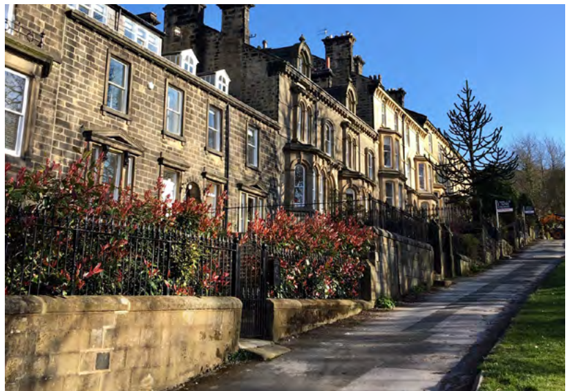
Typical boundary treatments include a combination of a low stone wall and railings. (Photo © Bradford Civic Society)
