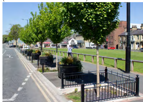
To maximise the value of new planting, these tree pits along North Street, Keighley, are designed as stormwater attenuation and treatment pits. (Photo © GreenBlue Urban)
